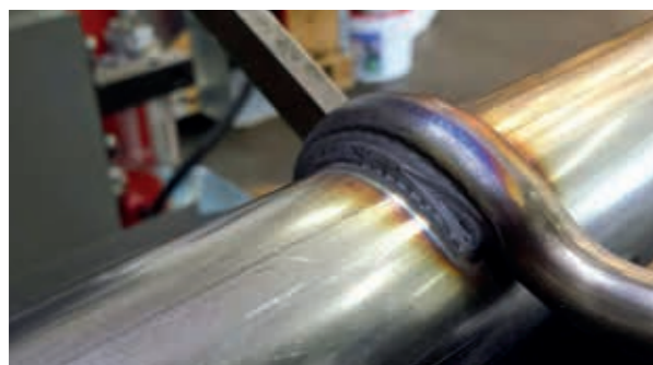
HD-MAG welding process
