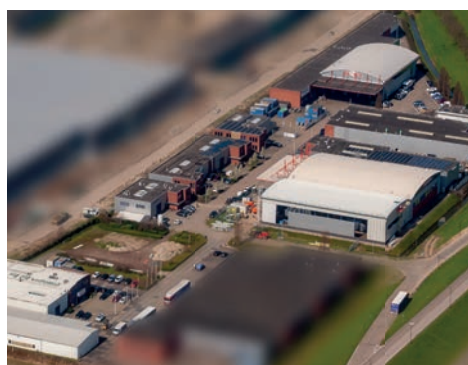
Valk Welding NL
